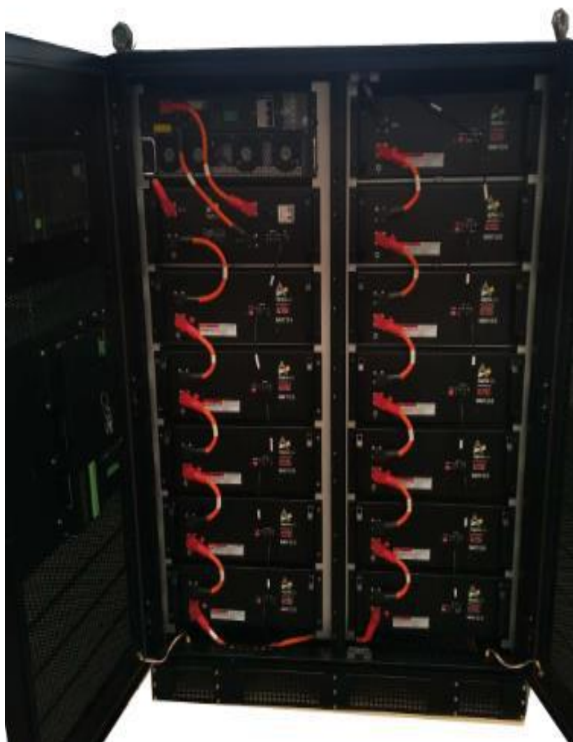
Figure 4.15 Completed installation of T30 System
